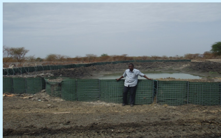
New fenced Oxidation Pond
